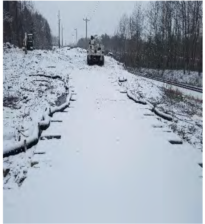
Fig 22: Filter sock installed on access road through wetland DW93. Viewing north. (12-17-19).
