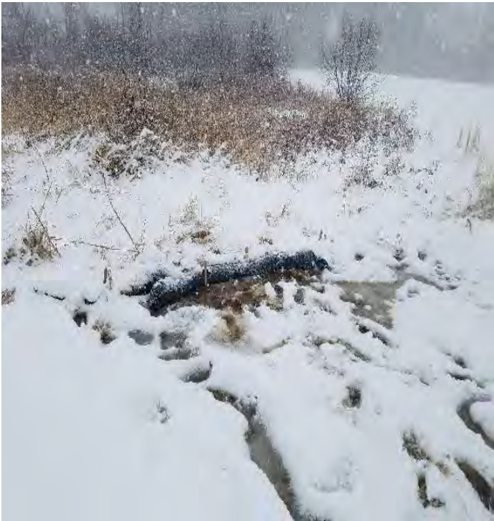
Fig 23: Filter sock repaired in wetland NW18 at Frink farm. Viewing north. (12-17-19).
