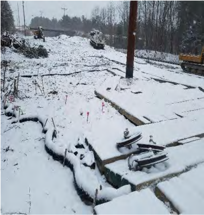
Fig 21: Filter sock installed around Str. 8. Viewing north. (12-17-19).
