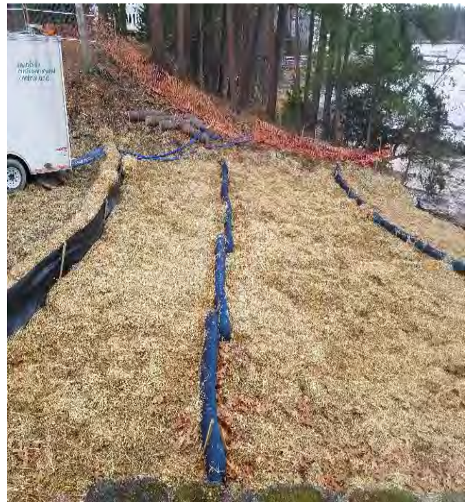
Fig 12: Sediment controls at Gundalow landing/east side of the Bay. Viewing south. (12-15-19).
