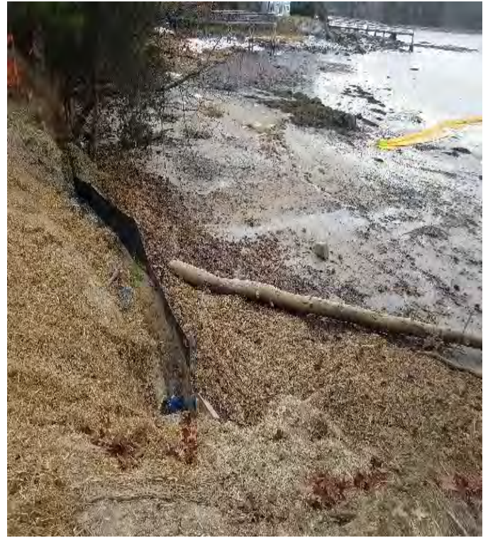
Fig 14: Sediment build up behind silt fence removed at Gundalow landing/east side of the Bay. Viewing south. (12-16-19).
