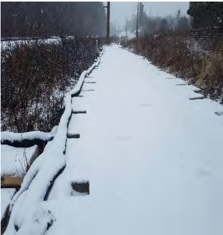
Fig 19: Filter sock installed along access road to Str. 3. Viewing south. (12-17-19).
