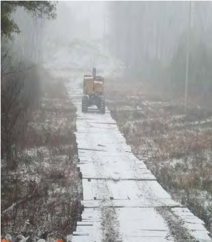
Fig 17: Building access road through wetland DW33. Viewing northeast. (12-17-19).
