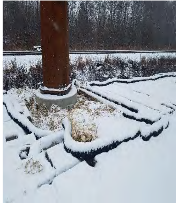
Fig 18: Filter sock installed around Str. 1. Viewing southeast. (12-17-19).
